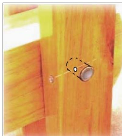
White line shows approximate nail position for attaching the pivot pin, through the wood.
